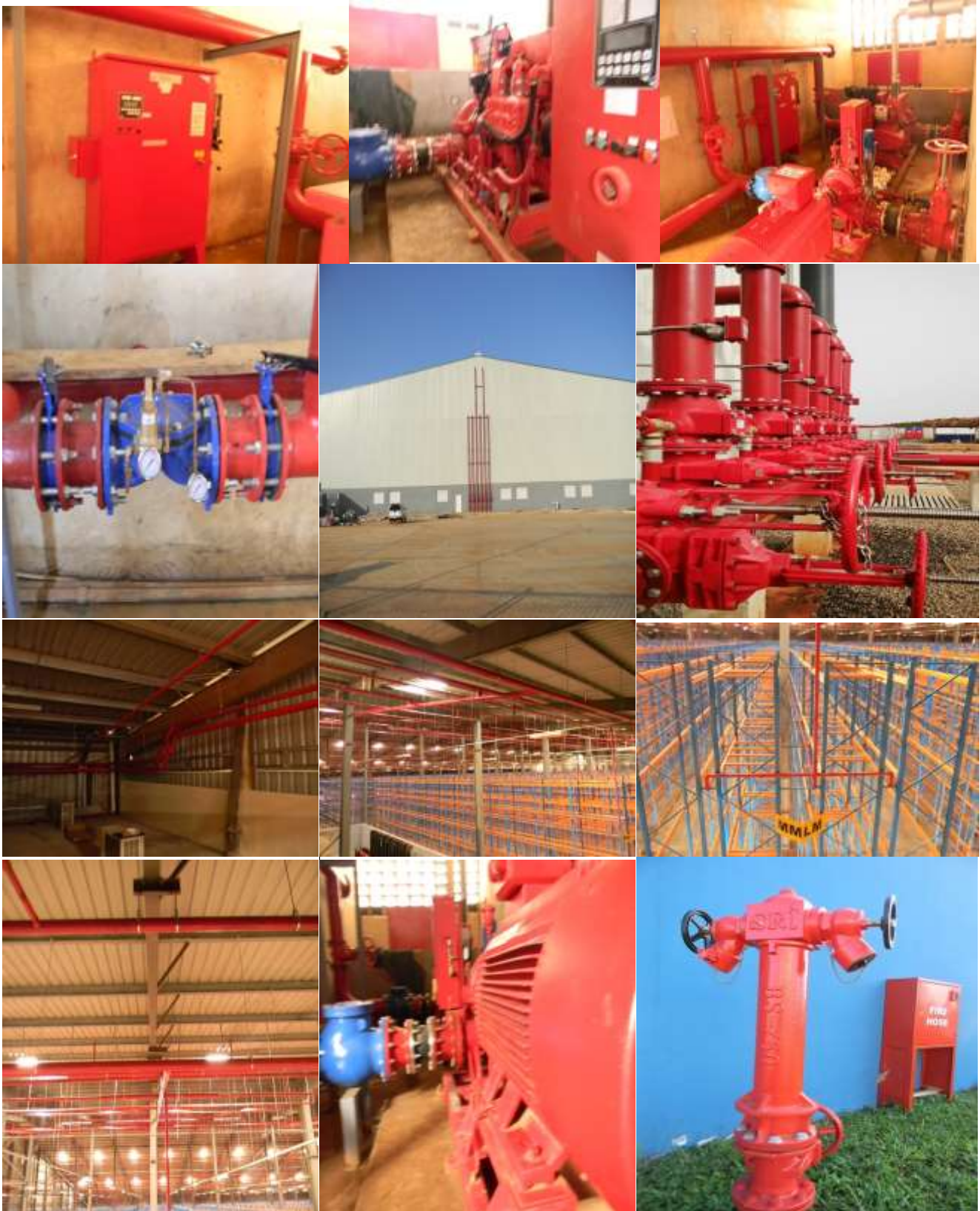
UNILEVER NIG PLC MEGA DISTRIBUTION CENTRE: FIRE FIGHTING SYSTEMS SHOWING HYDRANT & SPRINKLERS (ROOF SPRINKLERS AND IN-RACK SPRINKLERS.) 2012-2013-DESIGN & SUPERVISION OF THE FIRE FIGHTING SERVICES
