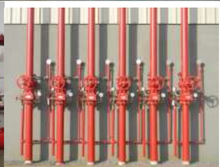
UNILEVER NIG PLC MEGA DISTRIBUTION CENTRE: FIRE FIGHTING SYSTEMS SHOWING HYDRANT & SPRINKLERS (ROOF SPRINKLERS AND IN-RACK SPRINKLERS.) 2012-2013-DESIGN OF THE FIRE FIGHTING SERVICES AND MECHANICAL SERVICES
