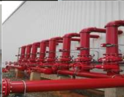
UNILEVER NIG PLC MEGA DISTRIBUTION CENTRE: FIRE FIGHTING SYSTEMS SHOWING HYDRANT & SPRINKLERS (ROOF SPRINKLERS AND IN-RACK SPRINKLERS.) 2012-2013-DESIGN OF THE FIRE FIGHTING SERVICES AND MECHANICAL SERVICES
